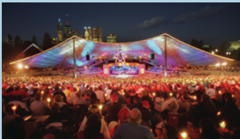
Figure sm.11 Band shells are used in outdoor auditoriums to reflect the sound waves towards the audience.
